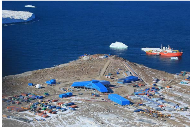
Figure 2 Jang Bogo Station in Terra Nova Bay
